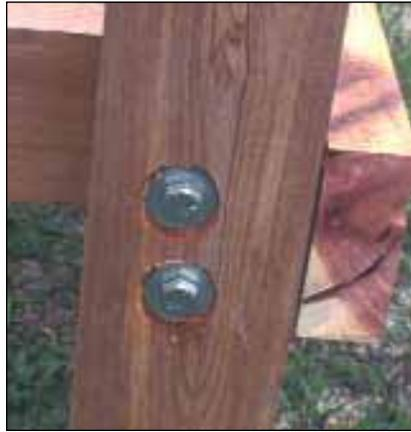
*Above left, if bolts are to be used to assemble the framework, be sure the exposed threads are positioned to the inside of the 4x4 posts. Right, for best appearance and to avoid accidental scraped legs, the bolt heads should be countersunk.*
